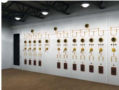
Adequate lighting for vertical surfaces, such as control panels, is important for keeping daily operations running smoothly – and critical in emergencies. Follow your lighting system's maintenance requirements, which will depend on light source and location. Photos: Holophane
